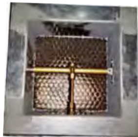
Airtech airflow measuring station with honey comb flow straightener
