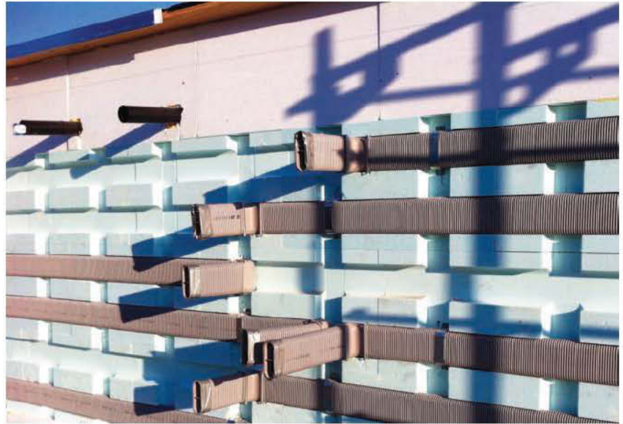
Multi-functional façade element with thermal insulation boards made of polystyrene (EPS) and integrated duct system made of polyethylene (HDPE) ©Fraunhofer ISE
