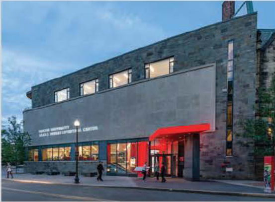
With VRF, a more dramatic look was possible without compromising the original building's architecture...
