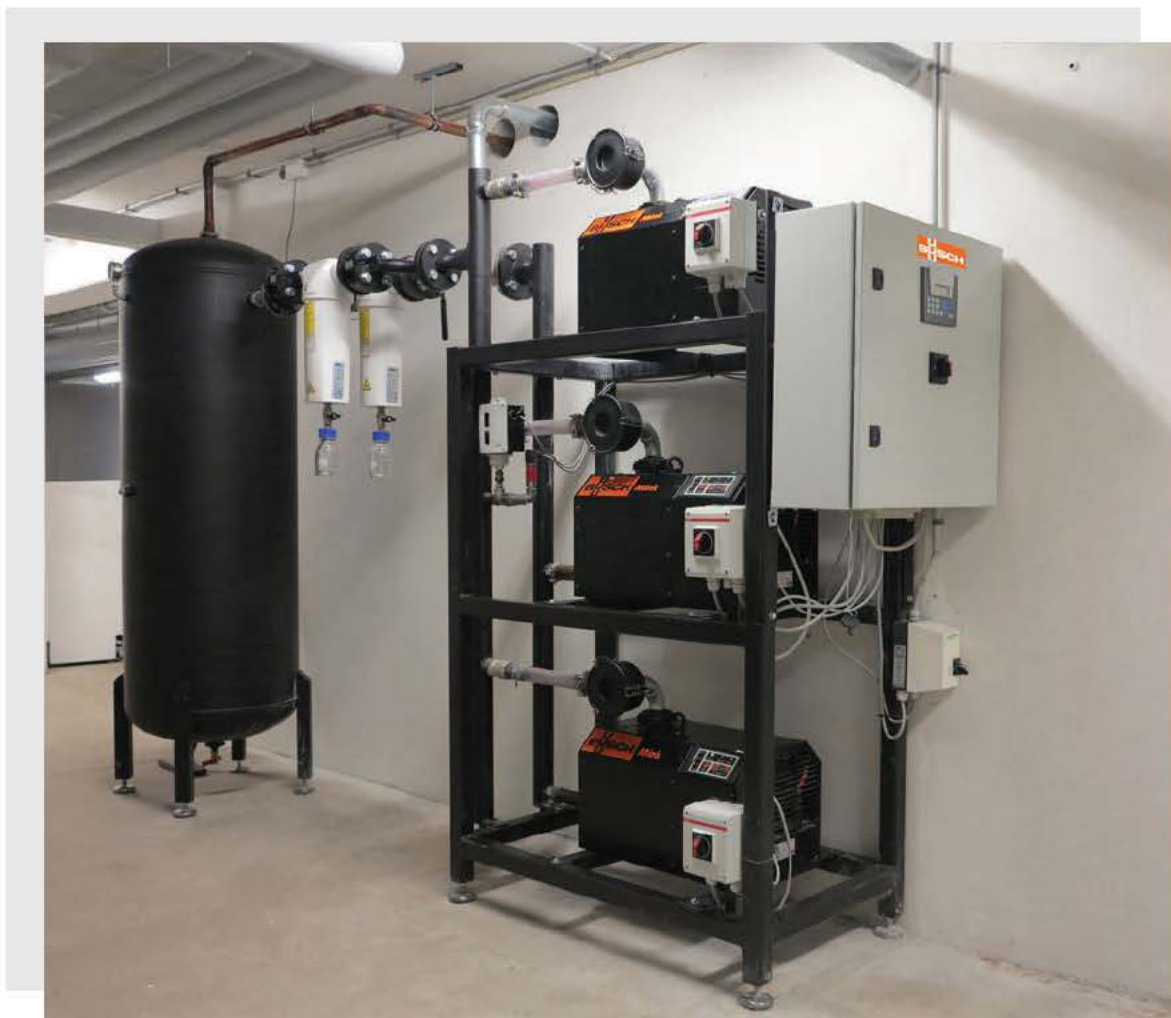
The VCR Viborg central vacuum supply with three Busch Mink MV claw vacuum pumps...
