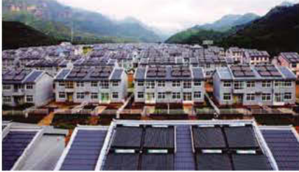
Solar water heaters being used in township in Northern China...
