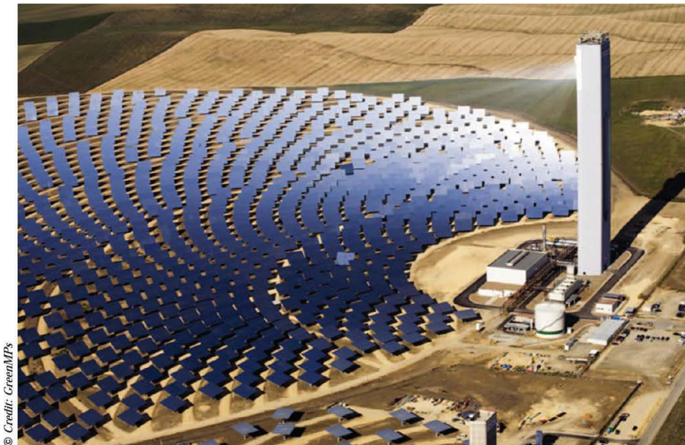
A sea of mirrors directs a powerful beam of light toward a solar power tower...
