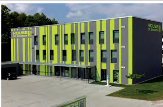
The project was developed by the building services company Airoptima, which now has its headquarters in the world's first Passive House Premium...
