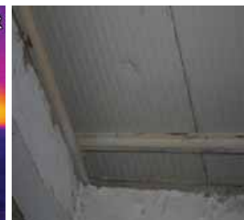
Leaks in the insulation material covering the cold storage unit can be a threat to the temperature uniformity inside the unit.
