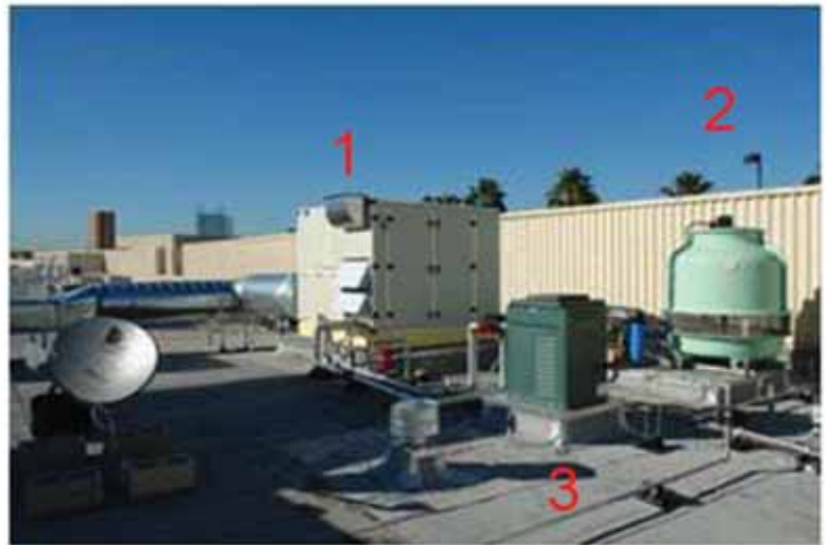
Figure 2: Major components and packaging of the AIR LDAC (Photograph shows packaged HMXs, water heater and cooling tower) 1: Packaged HMX; 2. Heater; 3. Cooling Tower
