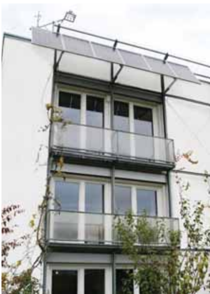
The building's two-part solar photovoltaic system covers 26 square metres and is mounted on the terrace as well as on the roof.
