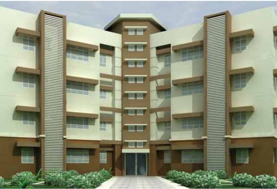
40-year old building was not air conditioned earlier as it was used as a staff quarter
