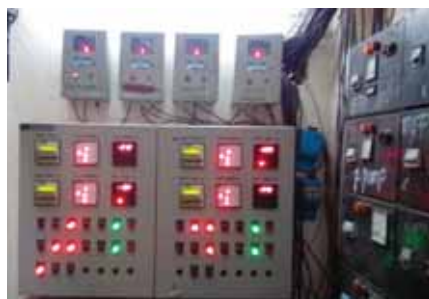
Automatic liquid level control, temperature control and hot gas defrosting system
