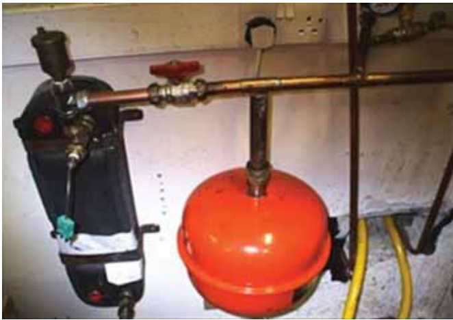
Figure 4: Shows the connections of the heat exchanger and expansion valve.
