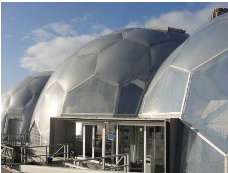
Floating Balls of Rotterdam cooled by Phase Change Material
