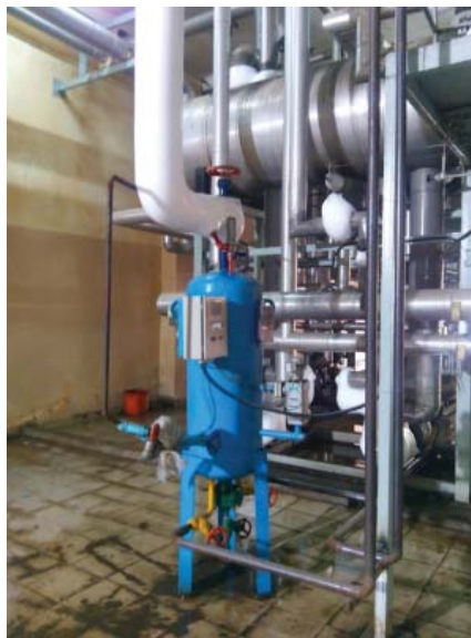
Figure 2: Ammonia Dehydrator Installation
