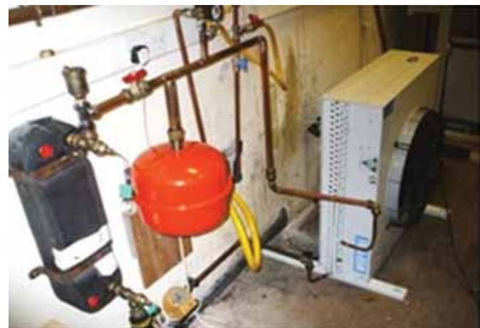
Figure 3: Shows the connections of the heat exchanger, water pump, heat rejection fan and expansion valve.
