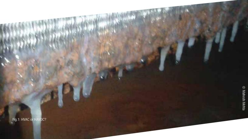
Deep coil cleaning may be done after, every three to five years for thick, hard working, dense coils, which are running continuously, should be cleaned intensely, or else it will start guzzling more power, spreading illness and giving cooling complain headaches...
