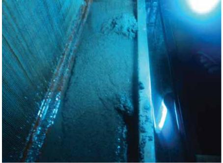
Figure 2: Cleaned Bio-Growth contamination residue in tray at another site. Avoid contamination spread, follow safety rules strictly...
