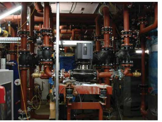
Flanged joints in a mechanical room: flanges are roughly twice the width of the pipe they are attached to...
