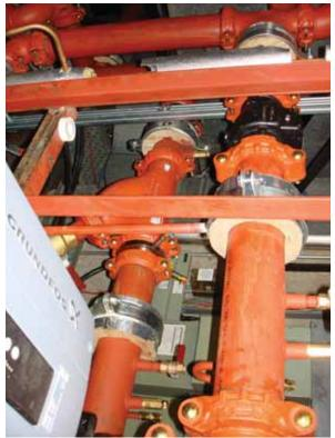
A mechanical coupling has 360-degree orientation capabilities and a low profile - making it ideal for installation in confined spaces...
