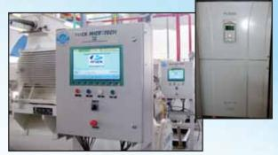
Frick India offers fully automated PLC controlled Refrigeration plant using VFD's.VFD maintain the suction pressure constant by continuously adapting the speed of the compressors. the main advantages are :
