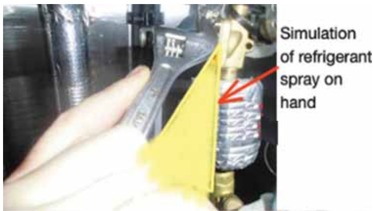
Figure 7: Simulation of Refrigerant spray on hand
