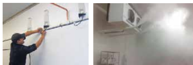
Figure 1.0 specially designed fogging head will put humidity only into the air, and not on the floor...
