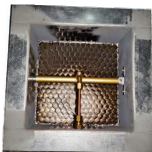
Airtech airflow measuring station with honey comb flow straighter
