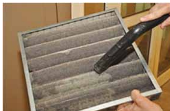
Figure 2. (above) A common air filter, being cleaned with a vacuum cleaner...
