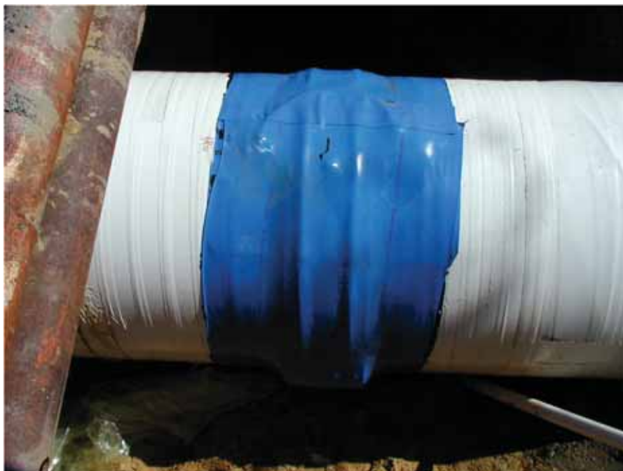
External coverings such as, heat shrink tubing, tapes or wraps, mastics, wax and asphaltic tapes may be applied directly over couplings...
