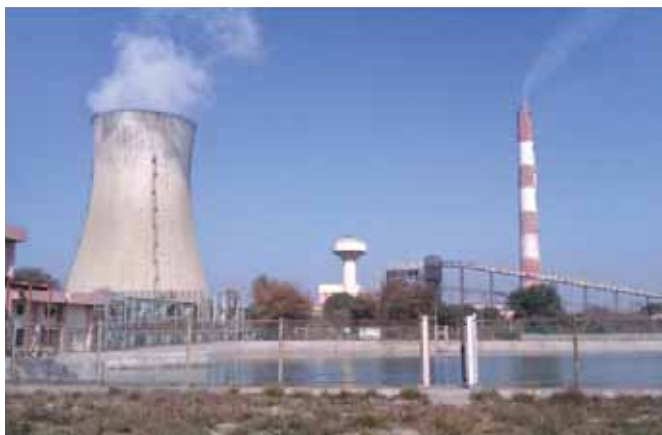
Figure 6: View of a natural draft cooling tower in operation...
