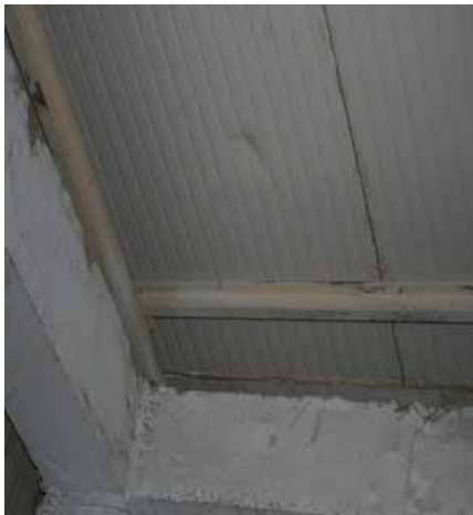
Leaks in the insulation material covering the cold storage unit can be a threat to the temperature uniformity inside the unit.
