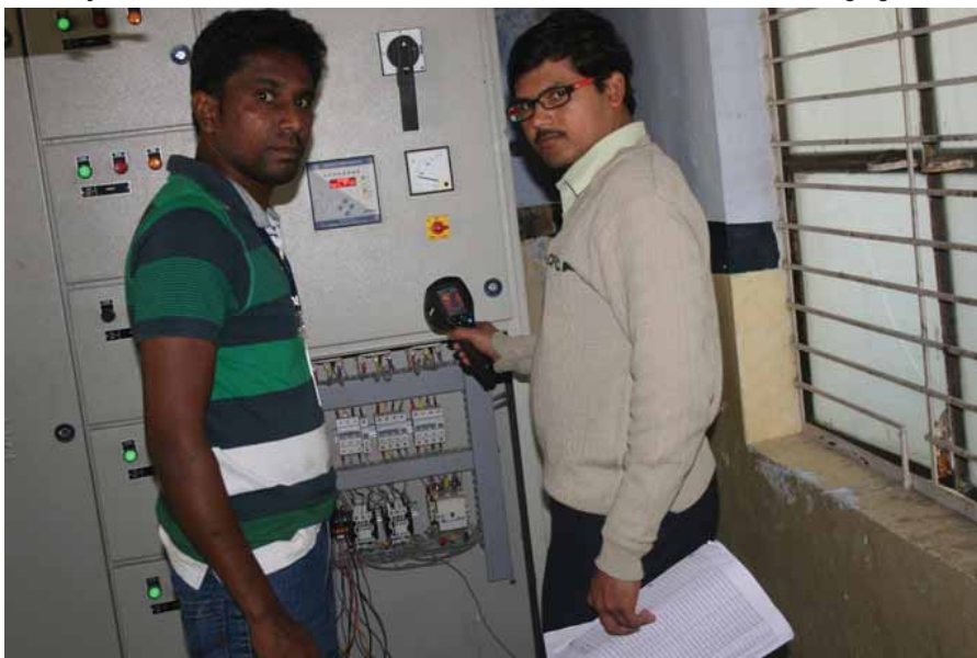
Gubba Group employees performing a thermal audit with FLIR i3 camera.
