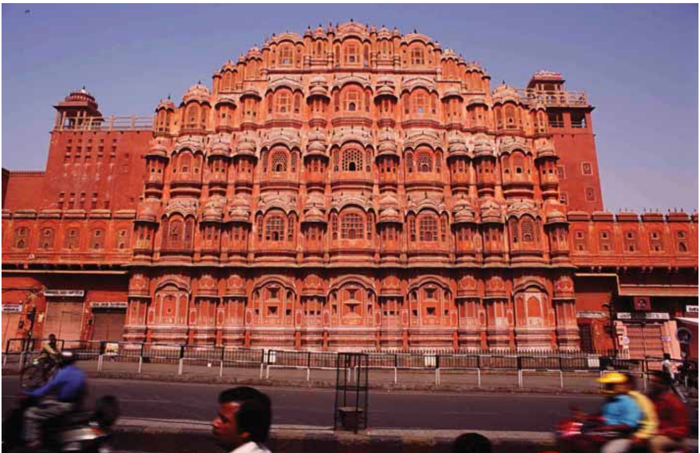
In the design of Hawa Mahals, the corridors are set in such a way to allow a high rate of air infiltration inside the building and ensure passive cooling in the same.
