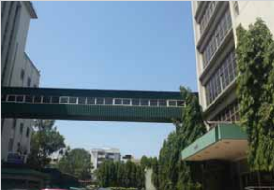
Carnac building has been the first establishment within Tata Power to get the Green Certification...
