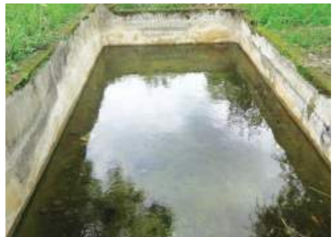
Fig. 1: Nocturnal cooling of the water the open tank
