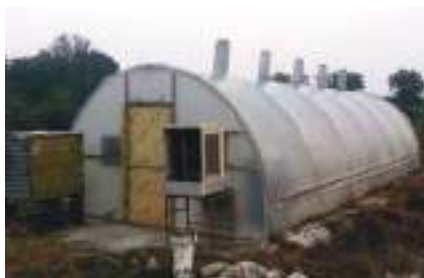
Fig. 3: View of solar drier fabricated for drying of fruits and Vegetables
