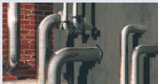
Piping Insulation
