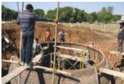
Fig. 3: Fixed dome type biogas plant under construction
