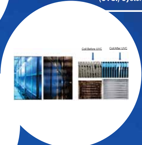
Ultraviolet Germicidal Irradiation (UVGI) System
