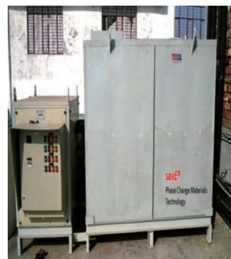
40 TRH flat plate TES system installation at Pluss
