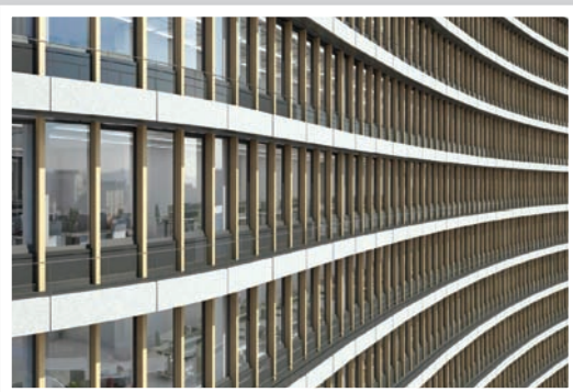
Up to a 1/4 th of the cost of cooling will be saved by the external blinds installed on all windows...
