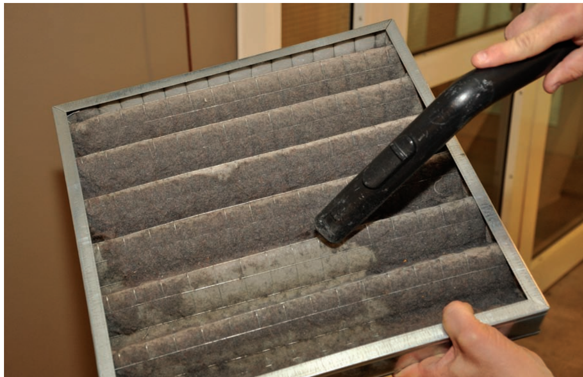
Fig. 2: A common air filter, being cleaned with a vacuum cleaner...
