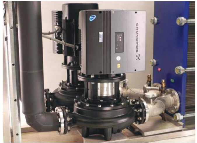
Grundfos TPE in-line pump, with built-in frequency converter
