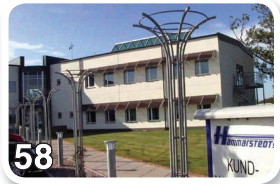
Building Insulation With Thermal Imaging
