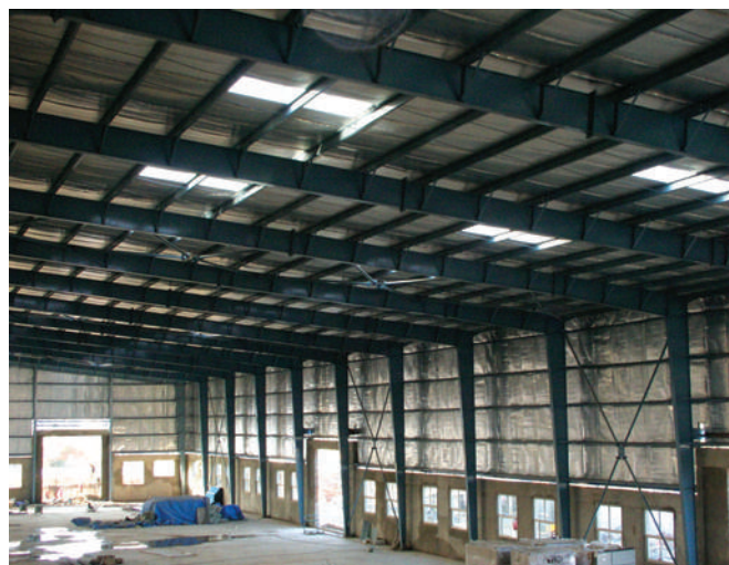
A reflective insulation system is typically formed by layers of aluminium or a low emittance material...
