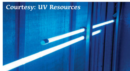
Fig. 6: Single-ended lamps can be overlapped...
